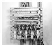
8. Label the cabling drop using the label identification holder and labels included, then insert the holder onto the wiring block. Use jumper wire or IC110 Patch Cords to complete the cross-connection.
