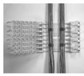
3. Route the cable within the base using cable/ VELCRO® ties with the tie down anchors to secure the cable.
