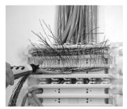
6. Position the conductors in the appropriate channel and trim the excess wire with a punch down tool.
