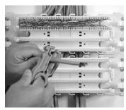
5. Strip back the cable sheath as much as necessary to expose the conductors for termination.
