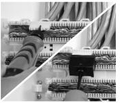
7. Align an IC110 Connecting Block in the proper channels of the wiring block with the blue mark towards the left and gray strip down. Use ICC's 5-pair or single punch down tool in the "HI Impact" setting to seat the connecting block.
