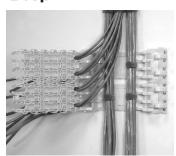
4. Feed the cables through the proper openings in the wiring block. Use cable ties with the tie down anchors on the wiring block to secure the cable. Close and latch the wiring block back into a secured position.
