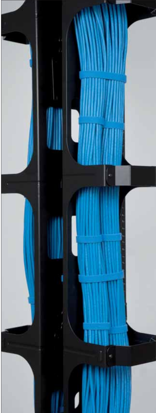
Mount on the front and rear of racks
