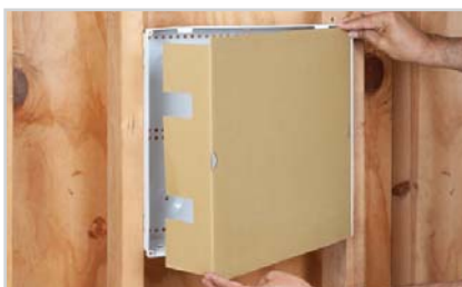
Mud guard to protect from the rough-in phase
